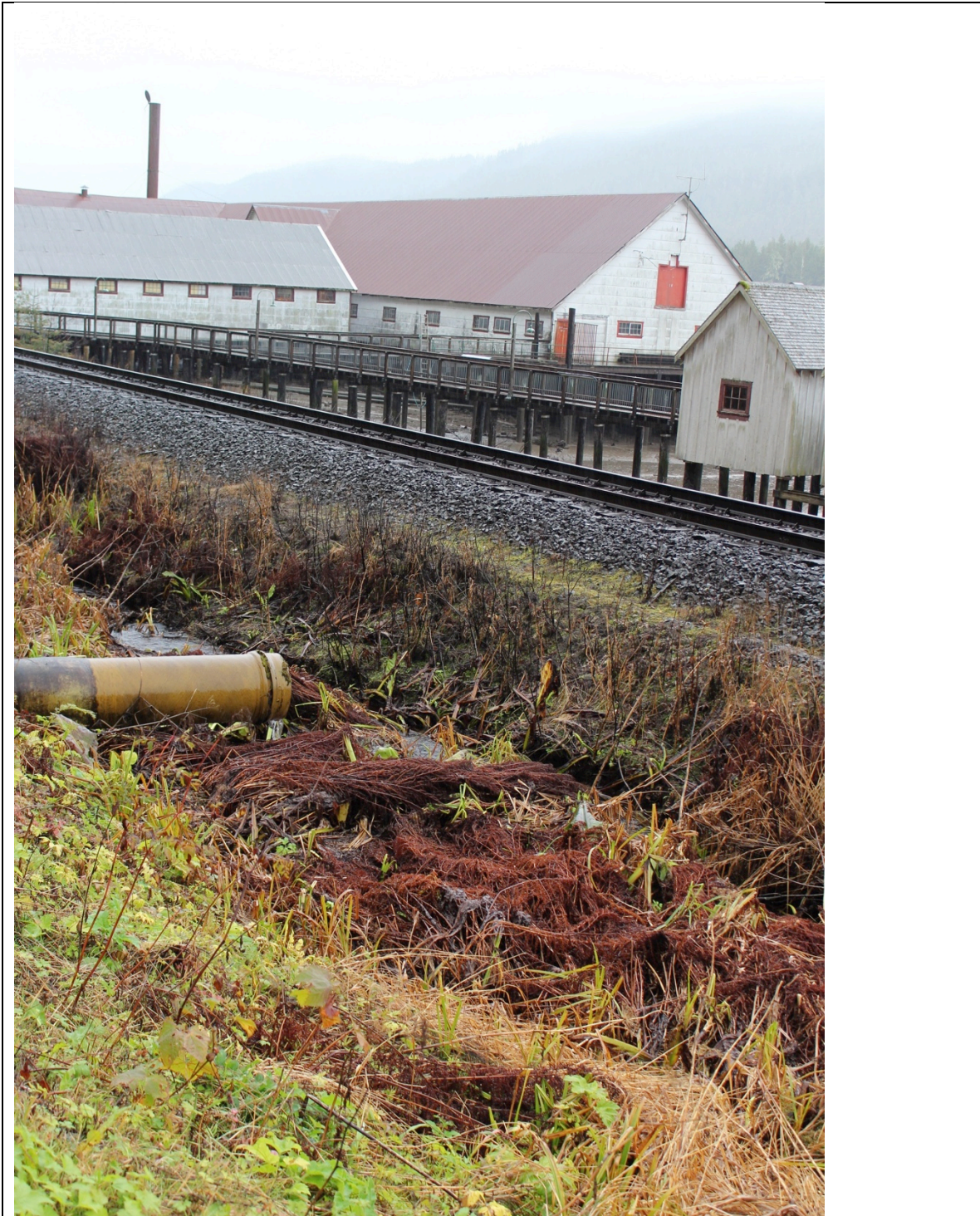
Photo 47. Downstream view of ditched channel with stormwater drain outlet.
